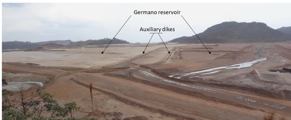
Fig. 17 Field picture of the auxiliary dike and the reservoir in the Germano mining complex.
