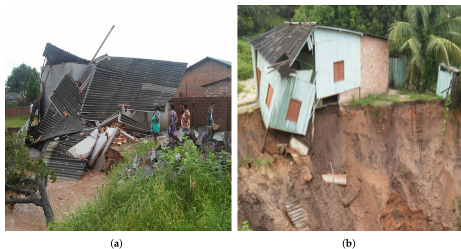
Figure 19. One of the municipalities affected by the extreme rain. (a) and (b) collapse of houses in municipality of Monte Alegre in Pará state. Photographs: Arney Barreto/G1 and Reprodução/TV Tapajós).
