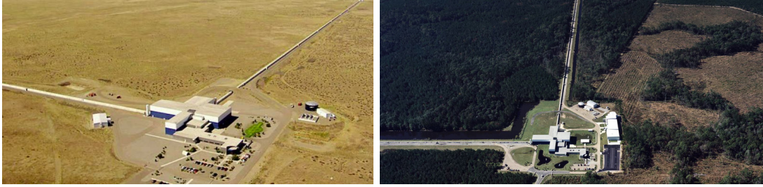
Figure 2.3 - The two LIGO sites: (left) Hanford, near Washington and (right) Livingston in Louisiana.
