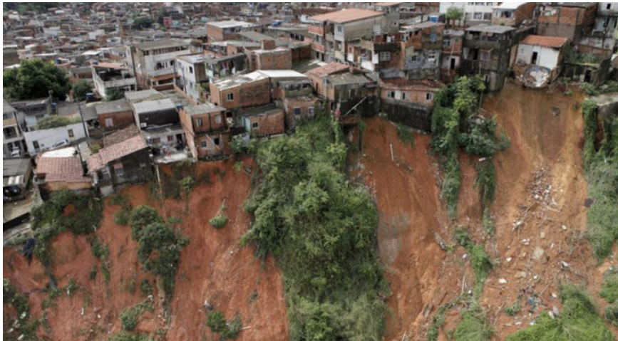
Figure 2.2 - Landslides at irregular occupation, Salvador (BA - Brazil).
