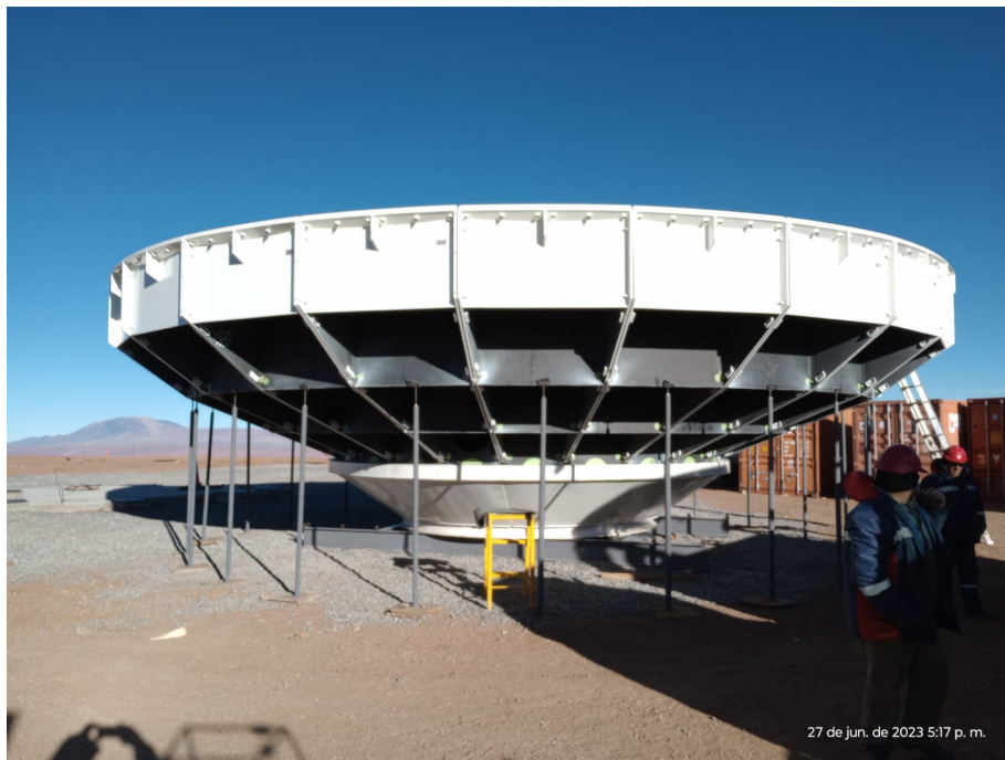
The dish of the LLAMA Radio Telescope being mounted.
