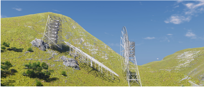
Fig. 1. BINGO telescope site – artist’s view. In this figure we show the hill and the use of the natural inclination of the terrain to place mirrors and horn structure. In this conception the control cabin is located under the service deck.
